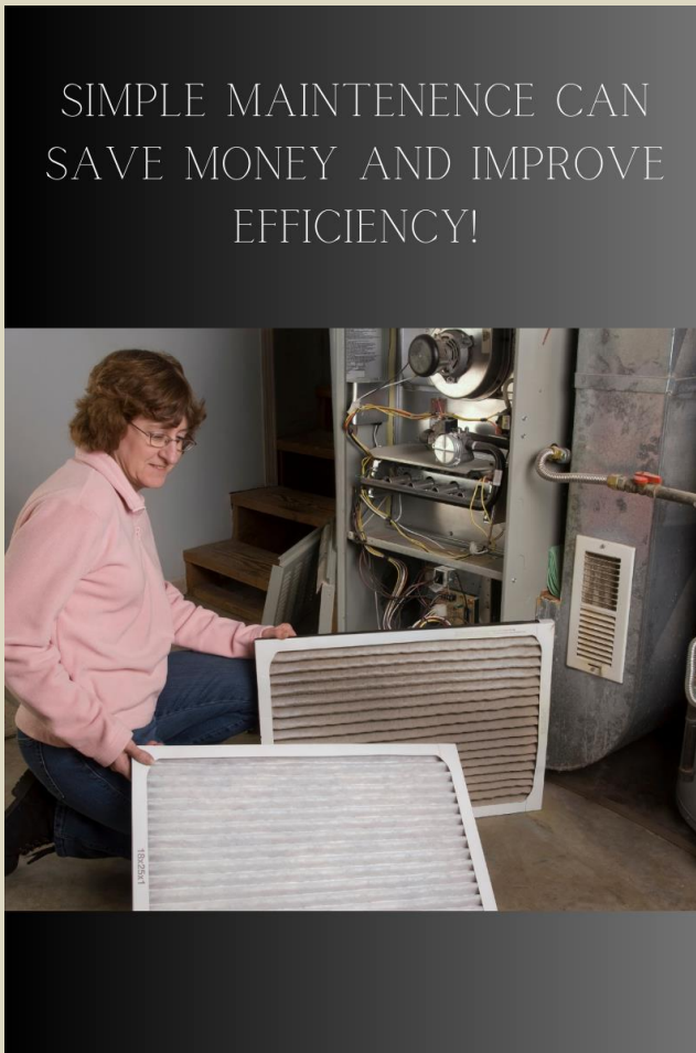
Regular change your HVAC filter to maintain its performance.
